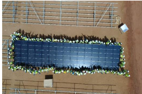
Solar power transforms IAMGOLD's Essakane mine
