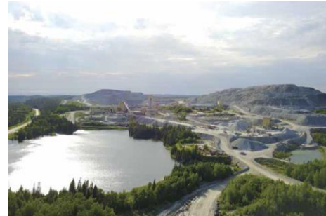
Award-winning optimised ventilation system at Barrick's Hemlo mine
